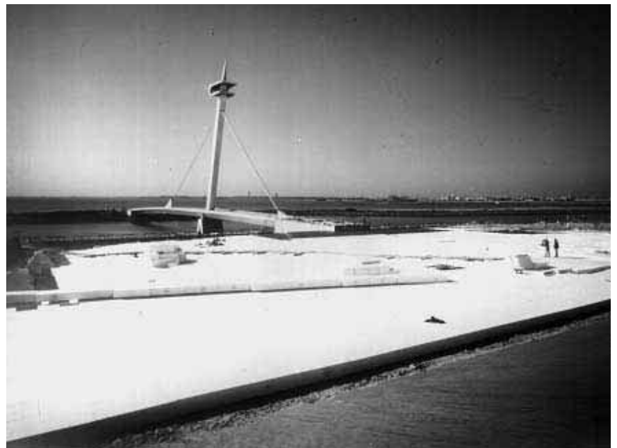
Fig. 14 EPS substructure (18000 m 3 ) at an abutment of the Kasai Nagisa Bridge, Tokio.
