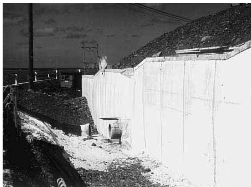
Fig. 12 Draining a steep-sided embankment.
