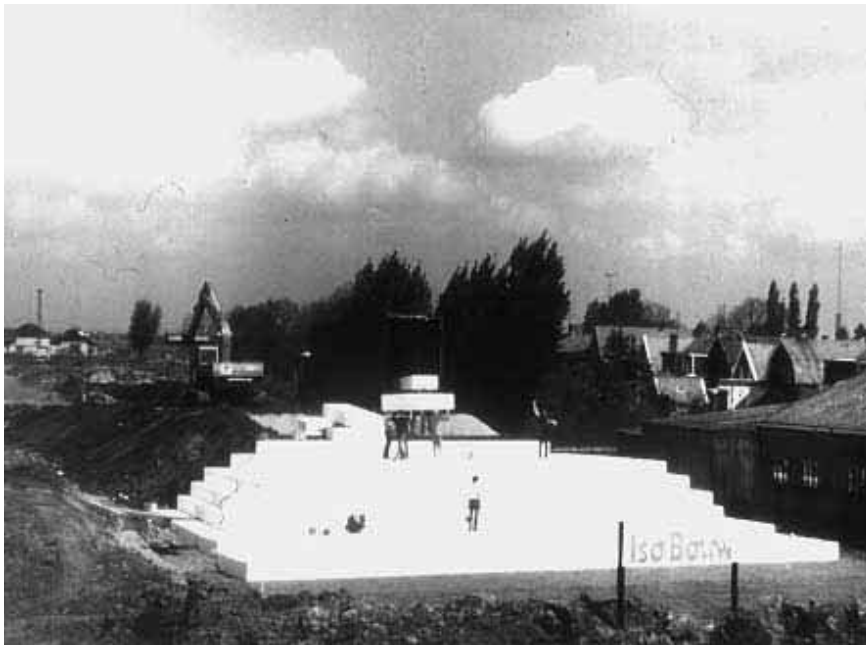
Fig. 5 Construction of an embankment using EPS (Hardinxveld-Giessendam, NL).
