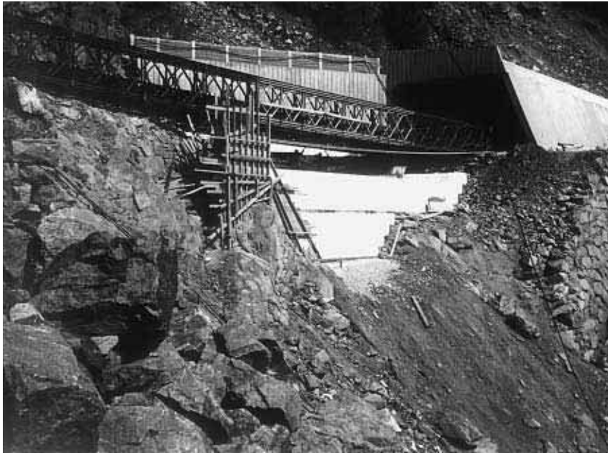
Fig. 13 Reconstructing a subsided mountainside road near Sougdahl in Norway using EPS.
