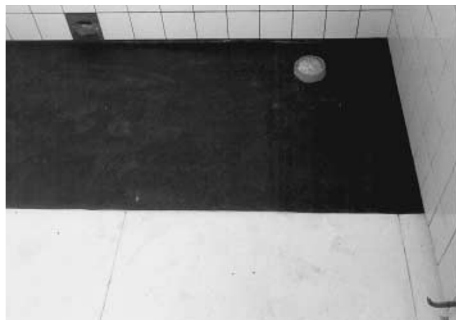
Fig. 8 Some of the insulating layer covered with bitumen felt
