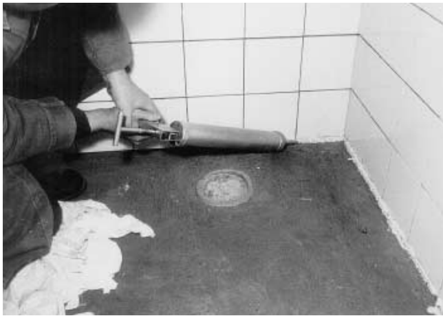
Fig. 10 Sealing the joints at the edges with an elastic sealant
