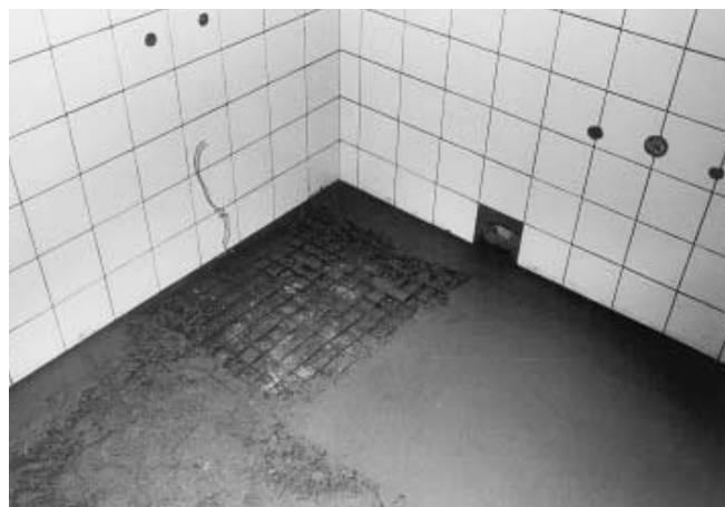
Fig. 9 Reinforced screed
