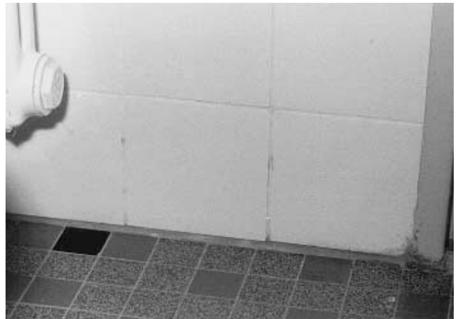
Fig. 13 Joint between wall and floor tiles filled with elastic sealant
