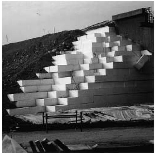
Fig. 7 Styropor blockware in the construction of causeways and bridge ramps in regions with poor load-bearing soils (European Highway E6, Ljungskile, Sweden).
