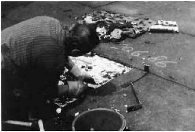
Fig. 1 Removing the roof covering to inspect Styropor foam panels that had been installed 31 years before. The joints between the panels were still tight.
